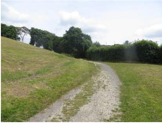
Plate 2.11: Deteriorating tarmac path leading west from Narberth
