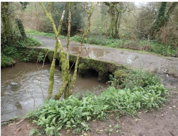
Plate 2.13: Bridge over Narberth Brook
